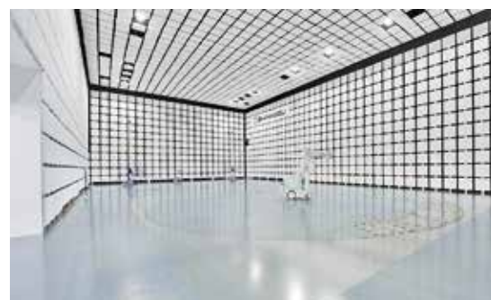
Anechoic Chamber at the Quality Center
