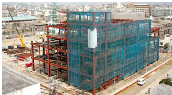
Construction of new analytical instruments plant (April 2006)
