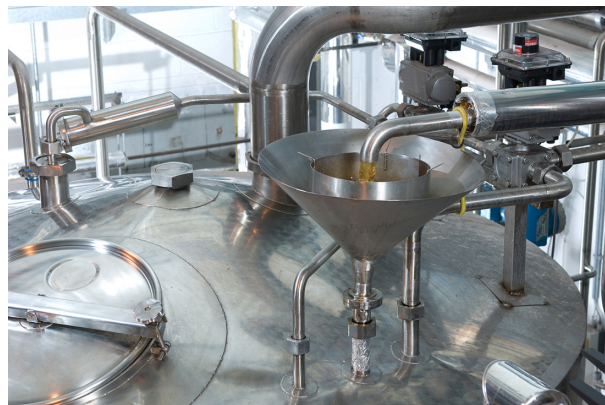
Fig. 2 Typical Food Production Equipment
