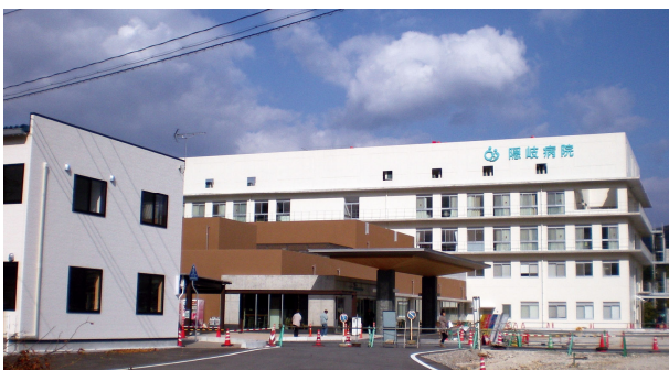
Fig. 1 View of Oki Hospital
