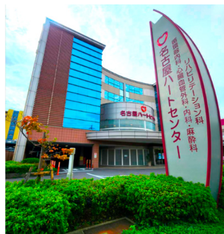
Fig. 1 Exterior of Nagoya Heart Center
