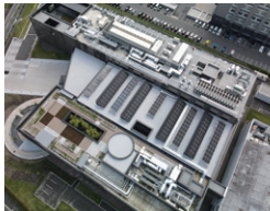
Using renewable energy
