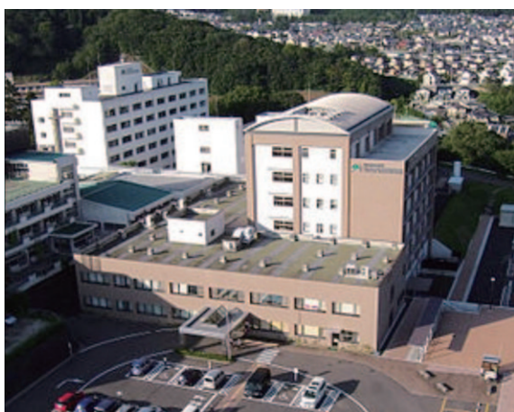
Fig.1 Exterior of Sendai Nishitaga Hospital
