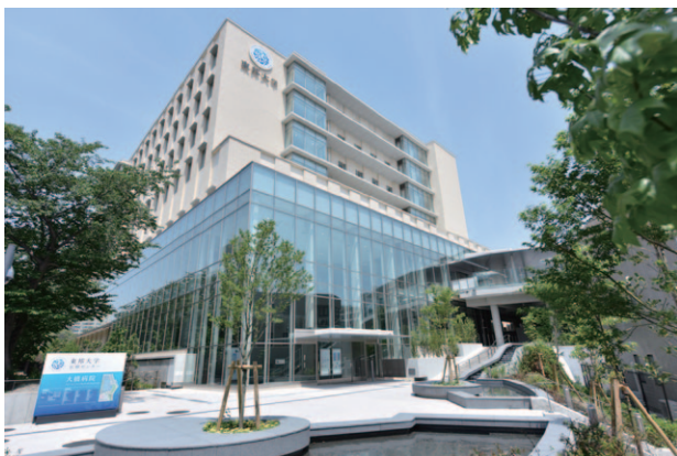
Fig.1 External Hospital View
