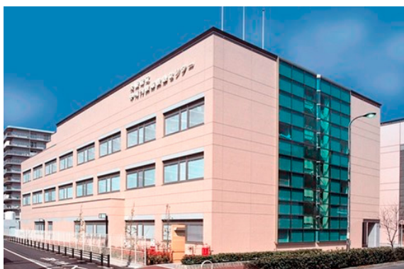
Osaka Prefectural Nakakawachi Emergency and Critical Care Center, the only tertiary emergency care center in the Nakakawachi medical district
