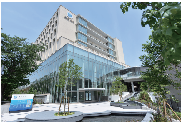
Fig.1 External Hospital View
