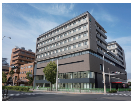
Fig.1 View of Imamura General Hospital
